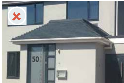
Unacceptable facade treatment
